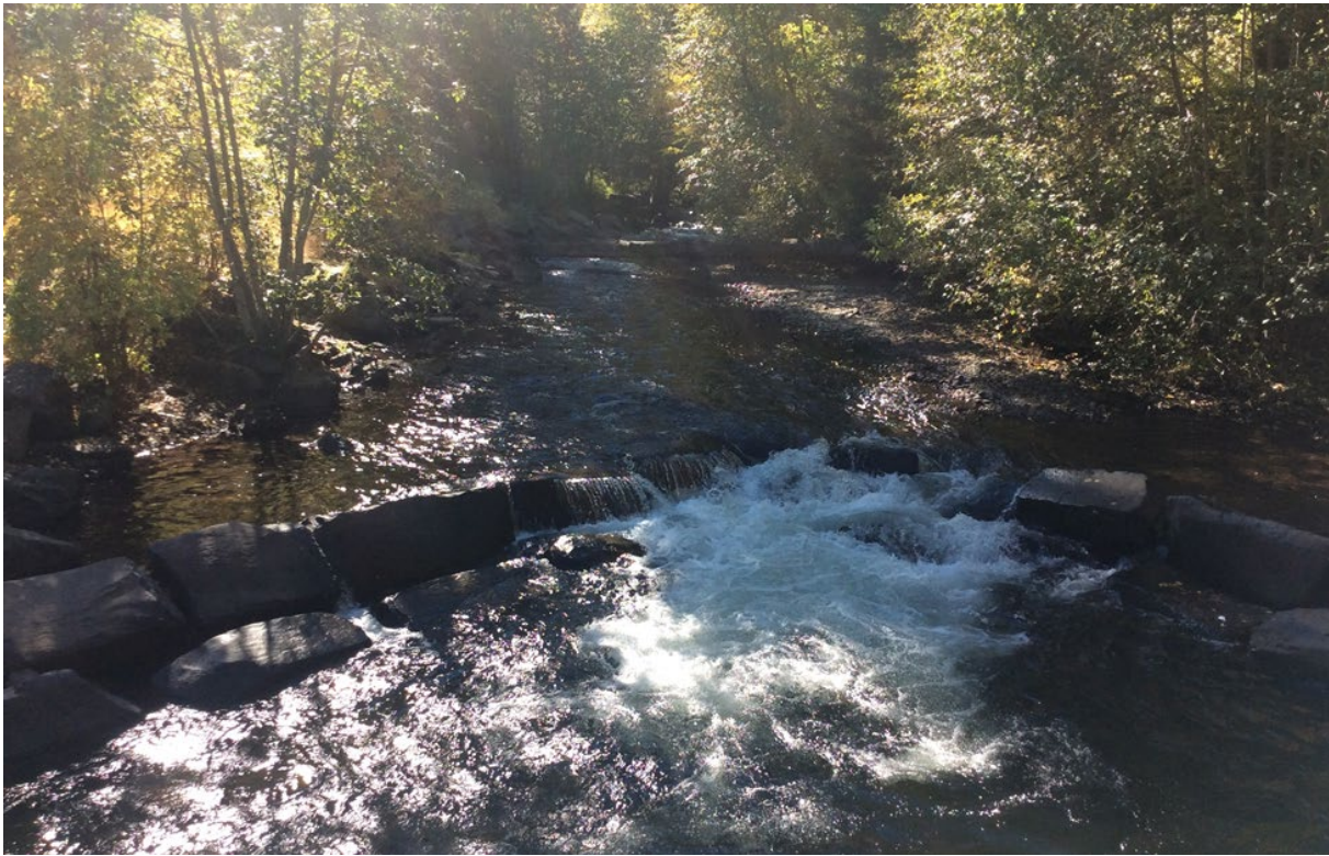
Figure 2-7 Rock Weir Restoration in Project Area 5
